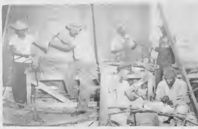
Principles of seamanapp are learned by members of the Marine School during their periods ashore. These men above, while waiting reassignment to lake tankers, get intensive training in various sea-going functions. These men are learning to splice wire. Training includes instruction in towing boats, sewing canvas, splicing slays and other wires, as well as training in safety and good housekeeping. As a result of the training, when the men return to sea they are better prepared to handle the problems that may come up.
